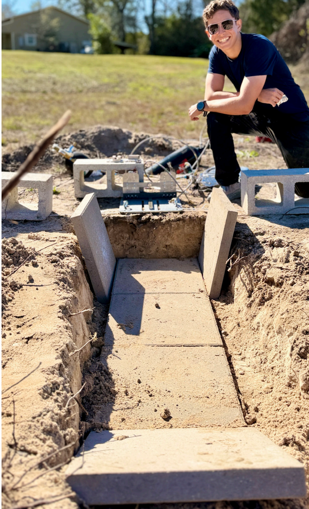
Test stand plumbing system (L) and exhaust plume trench (R)
